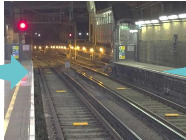
March '15 – Infrastructure installed to support testing in Central London
